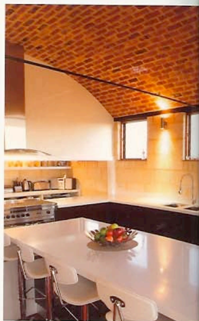
BARREL OF FUN: The unusual barrel-vaulted ceilings are recycled brick laid into steel frames - a feat of engineering that has attracted international attention. (below) The kitchen decor is minimal thanks to appliances hidden in a scullery behind.
